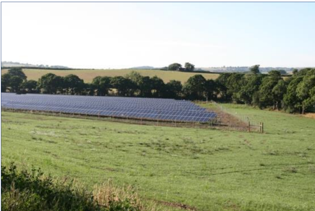
Figure 2.2: Example of a solar PV development near Crediton
